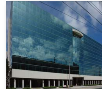
7000 Building South Miami, Florida
